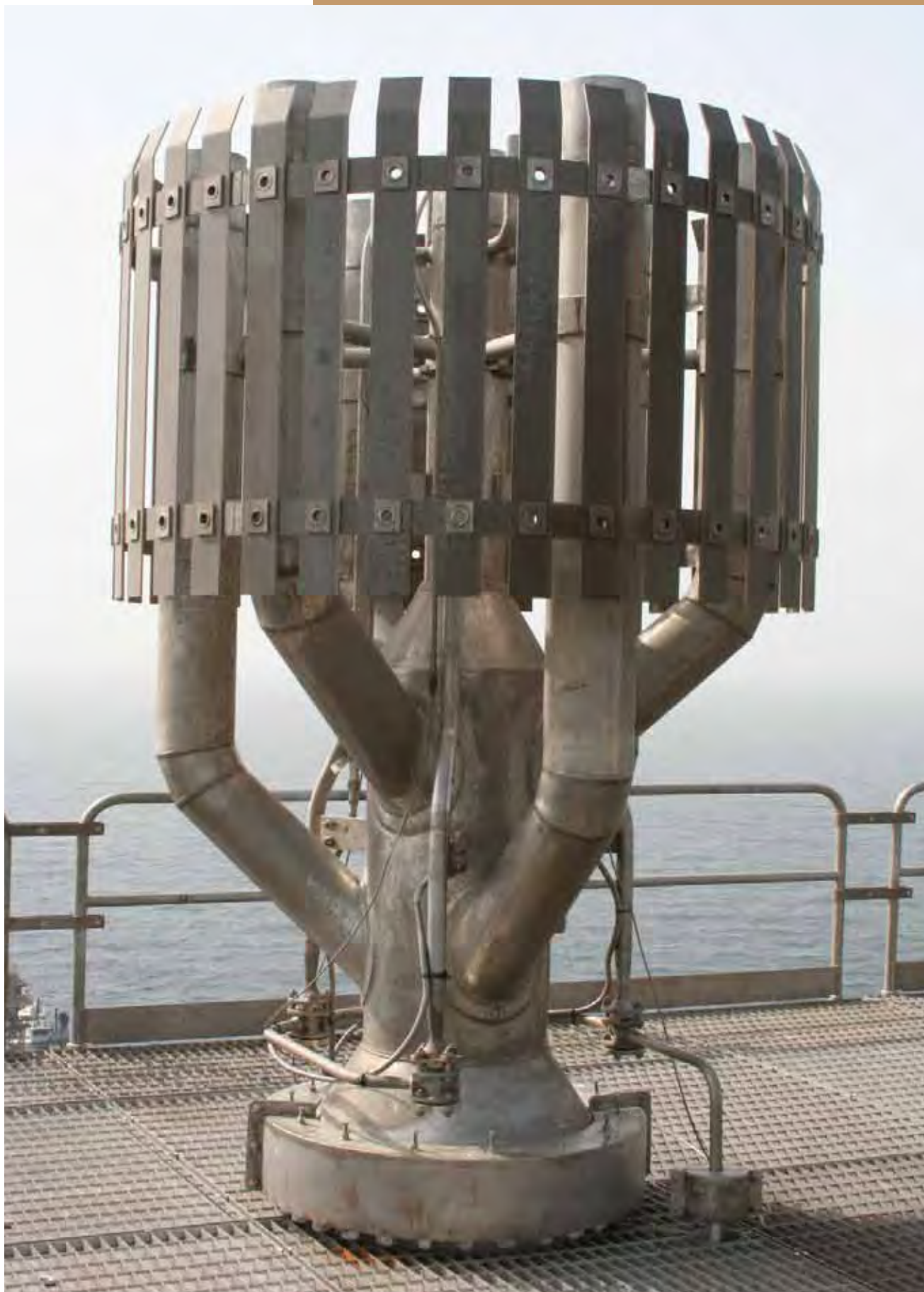
CSF-7-8 HP Flare Tip Offshore Qatar
