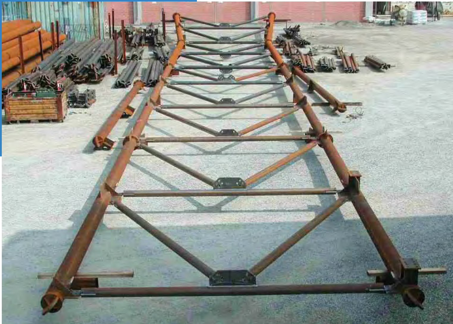
Trial Assembly of Derrick Structure
