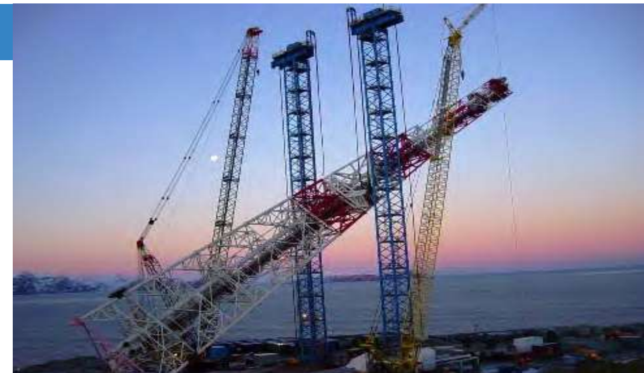
130m Derrick Structure single lift Hammerfest LNG project, Norway
