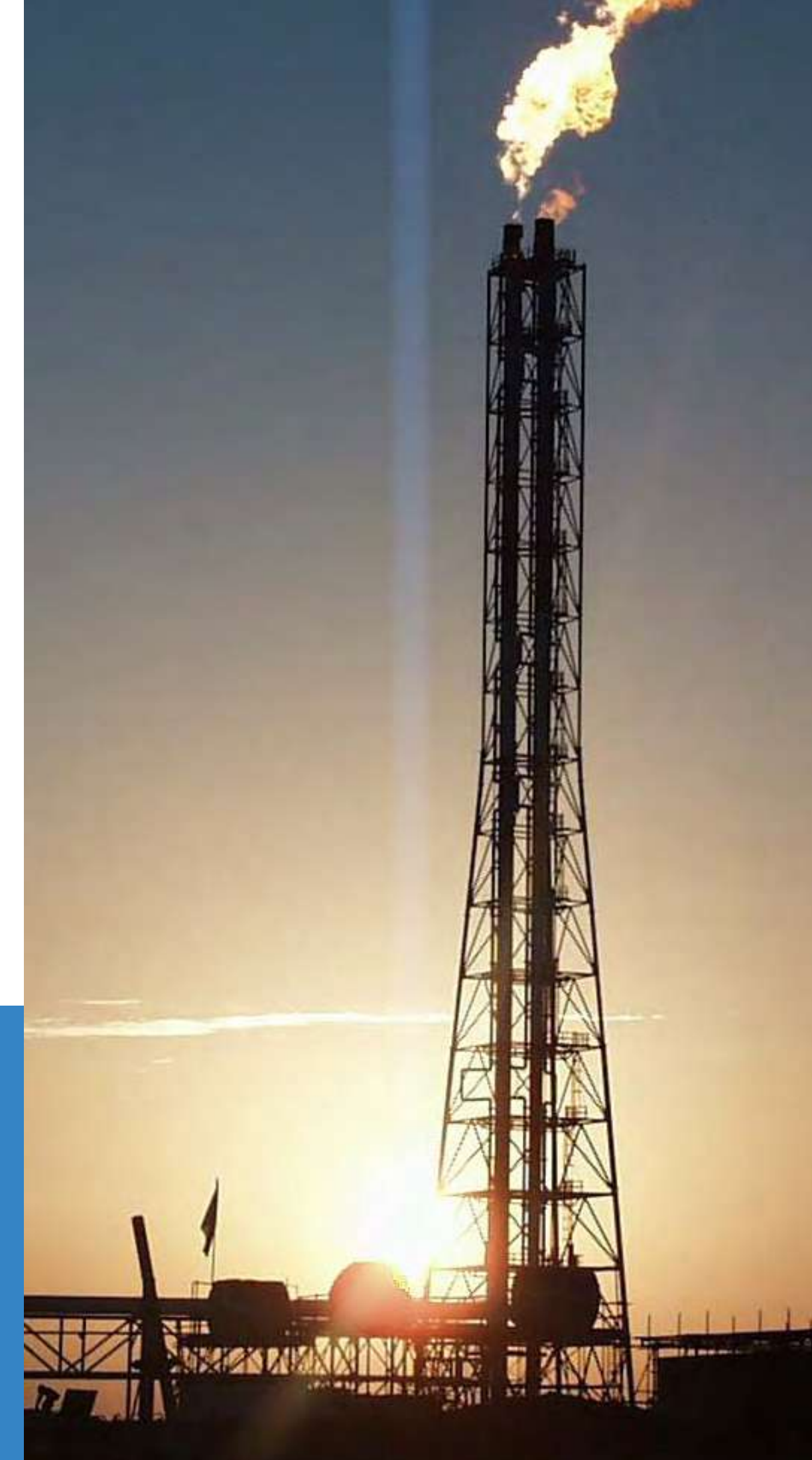
Derrick Supported Multi-flare System Ethylene Project in the UAE
