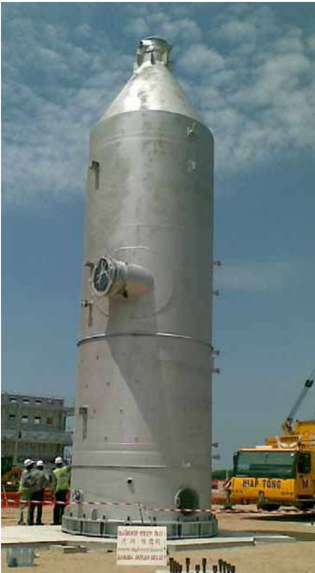
Vertical Knock-out Drum Refinery, Singapore
