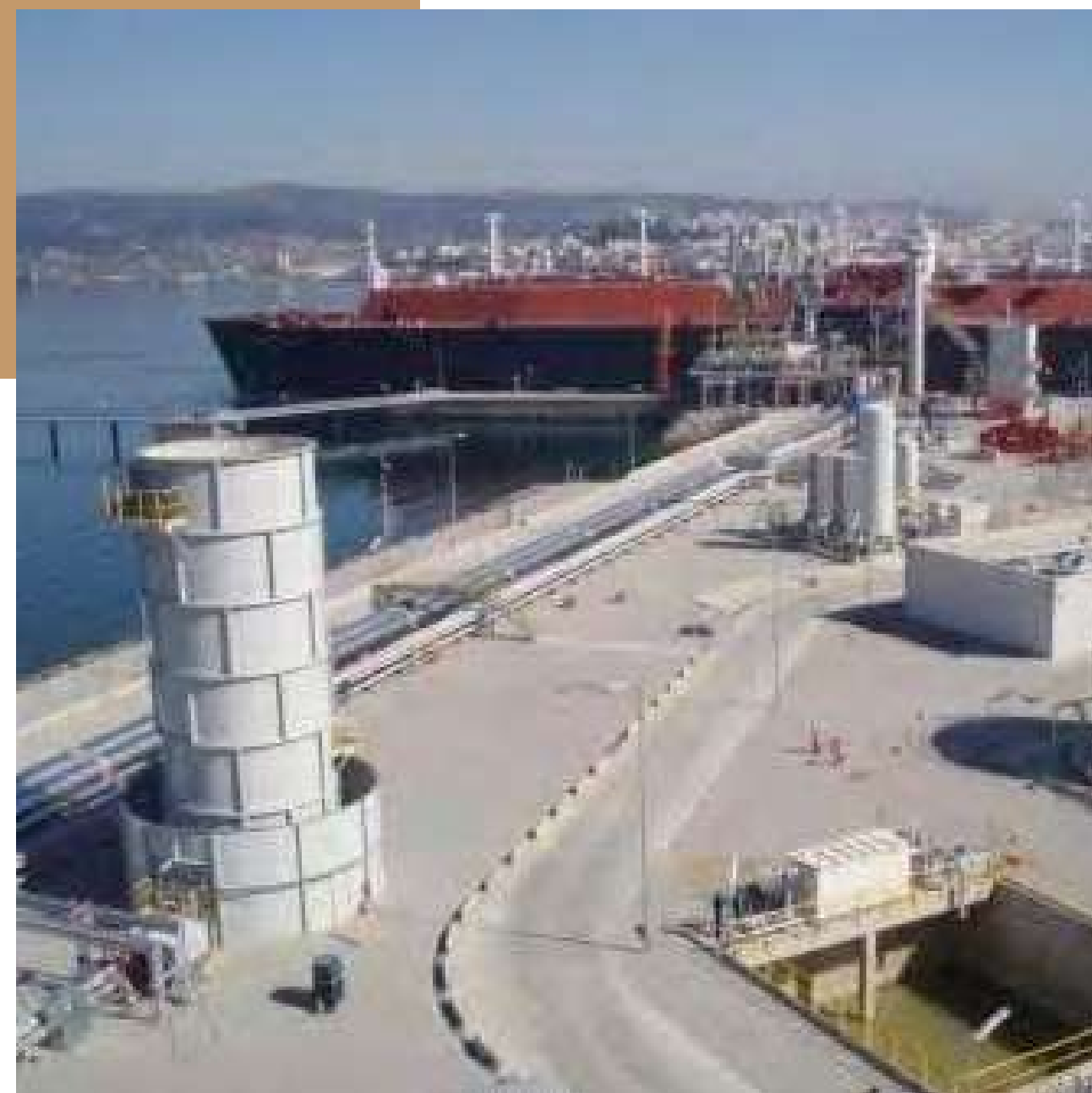
15t/h Enclosed Ground Flare Mugardos, Spain
